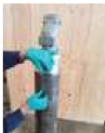
Slide joint section to remove screen from pump.
